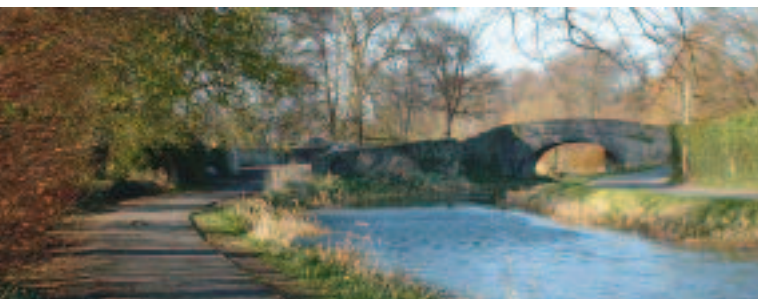
Tandys Bridge on the Canal
